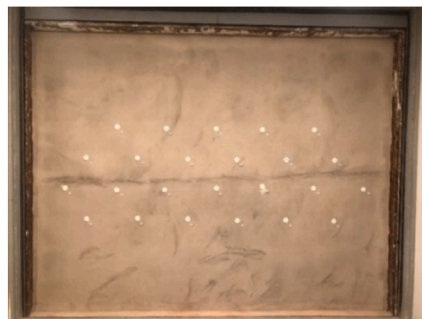
Fig. 5b. Stage 2: The 24 controlled openings of smaller holes.
