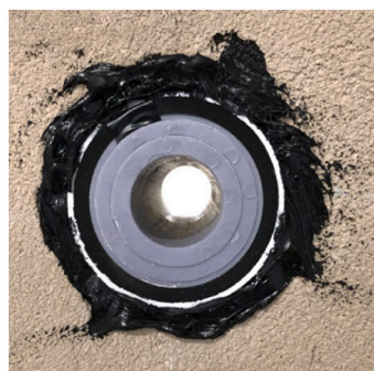
Fig. 6c. Stage 3: Large openings. Detail.
