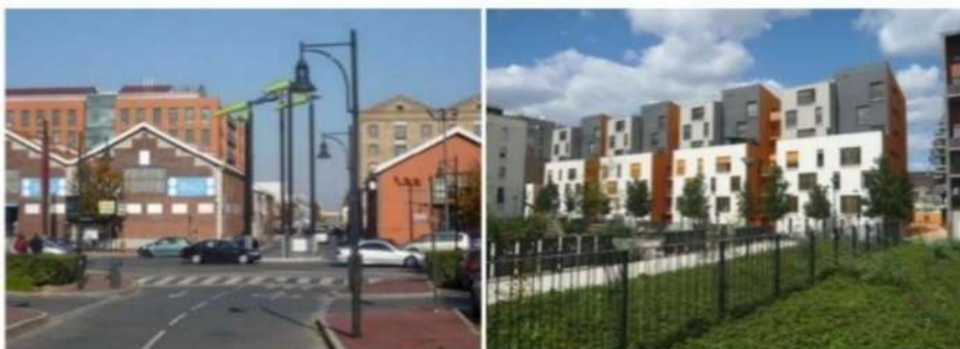
Fig. 16, South of La Plaine by Icade, a former warehouse sector has undergone new construction (left). new communal rental housing in the Montjoie neighborhood, centered on a plaza (right) [53].
