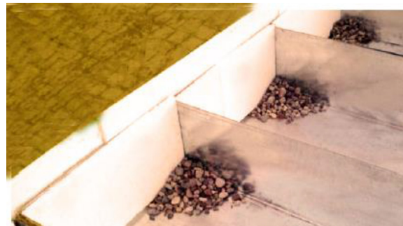
Fig. 5. The foam boards around containers and small aggregates at the drainage hole top (Author).
