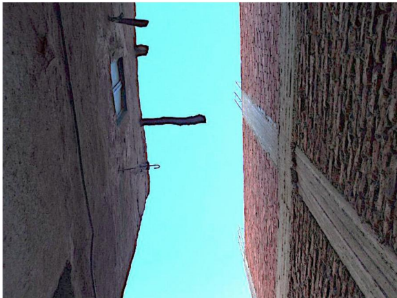
Figure4- 8 Mud brick house aside by a concrete house in Ghawassa village (Source: (ElMoeulhi, 2014)
