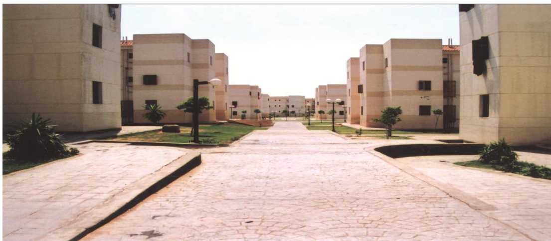
Figure3- 5 A view of Zenhum project after development (Red Crescent, 2011)
