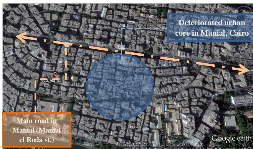
Figure2- 15 this fig. shows the Manial distict and the deteriorated urban pocket which is very near to the main road.source: (GoogleEarth,2016) edited by the Researcher
