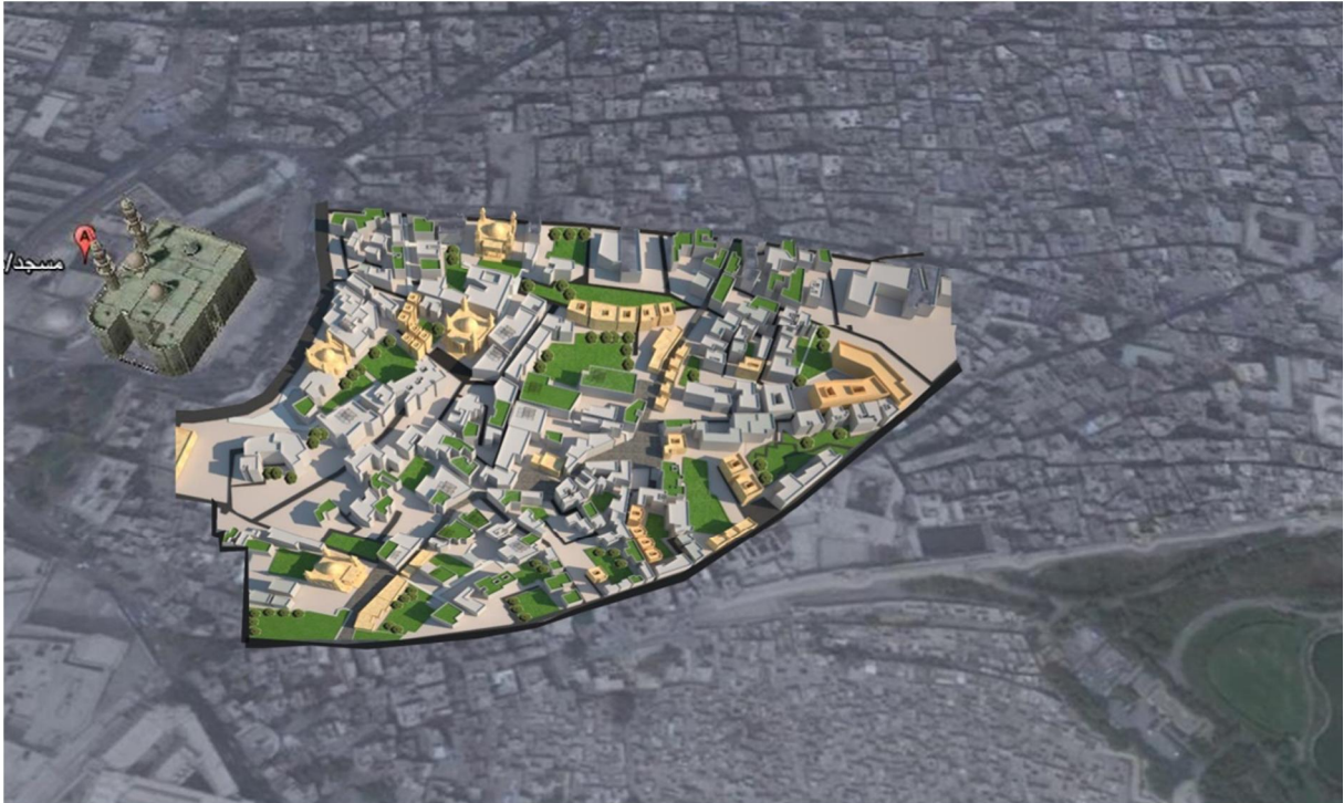
Figure7- 18 An aerial view showing the relation between the developed area of Darb El Labbana with the entire context (Researcher,2016)
